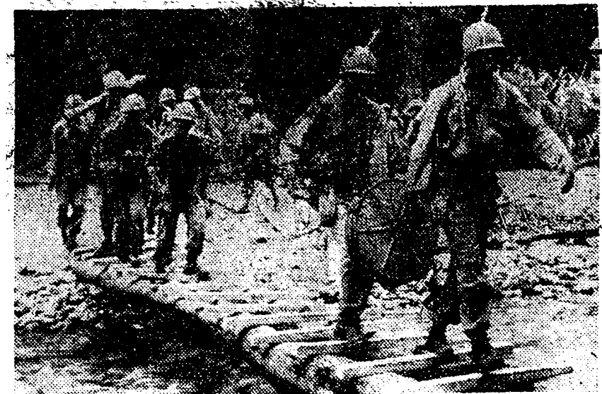
ENROUTE TO THE FRONT —The above photo shows something of the natural obstacles provided by jungle growth and rushing streams that the 93rd Division must conquer at Bougainville. Here a combat team crosses the Laruma River over a newly constructed bridge built by the engineers, carrying ammunition and supplies on their way to the front.
